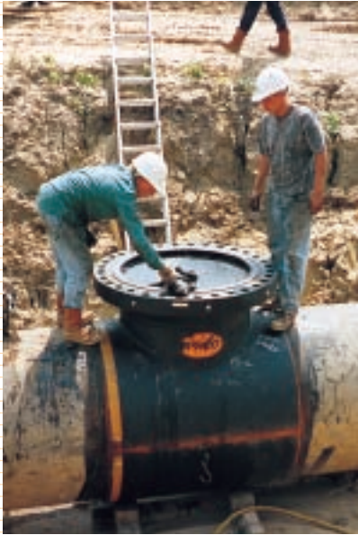
48" (1200mm) line stop fitting with completion plug installed on crude line.
