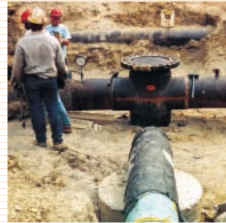
20" (500mm) Sure-stop bottom-out fitting with completion plug installed.
