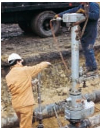
8" (200mm) hot tap line stop operation and 2" (50mm) equalisation tap.
