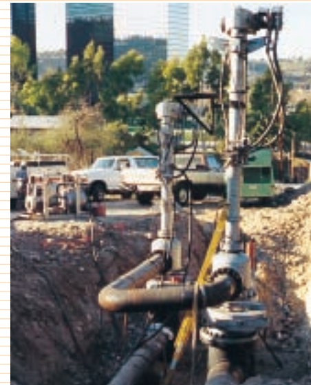
Double 20" (500mm) Sure-stop on natural gas line with 14" (350mm) bypass.
