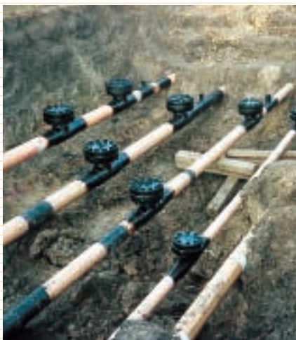
Line stop equalisation and bypass fittings for multiple line relocations.
