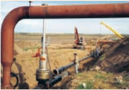
14" (350mm) line stop with bypass.
