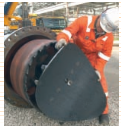
Removal of coupon.
