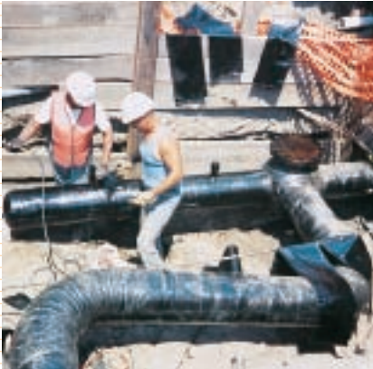
Spherical Tee line stop fitting with side outlet for permanent relocation.
