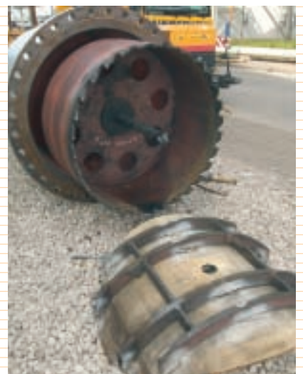
36" coupon showing bracing support.
